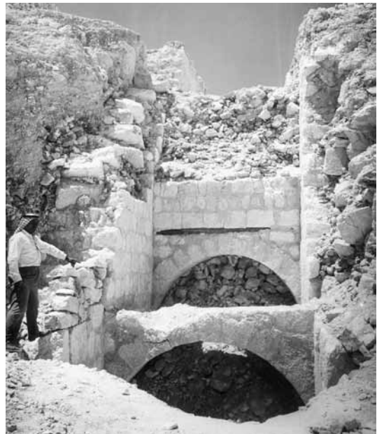
Fig. 2. Uppermost arches of the passageway as revealed during Foerster’s excavations (view from northeast) (© G. Foerster).
